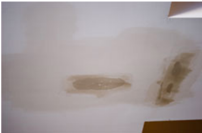
Figure 1: Water-stained drywall.
